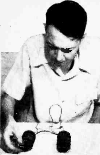
Author demonstrates how one Selsyn follows movement of mate.
